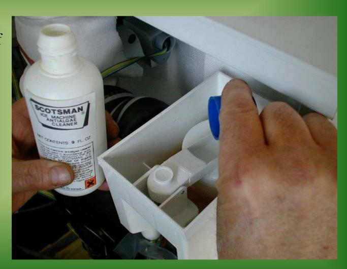
....place again thewater reservoircover payingattention to removethe jumper betweenthe two metal pins.
