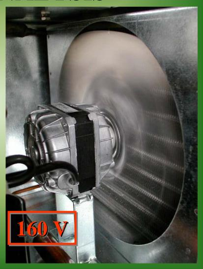
During normal operation mode the fan motor is energized at 230 V during its ON mode and.....
