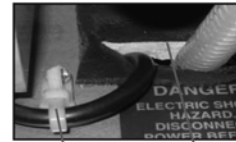
Cord Fastener Cutout in Pump Deck
