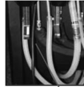
Route and up and behind Valve Panel
